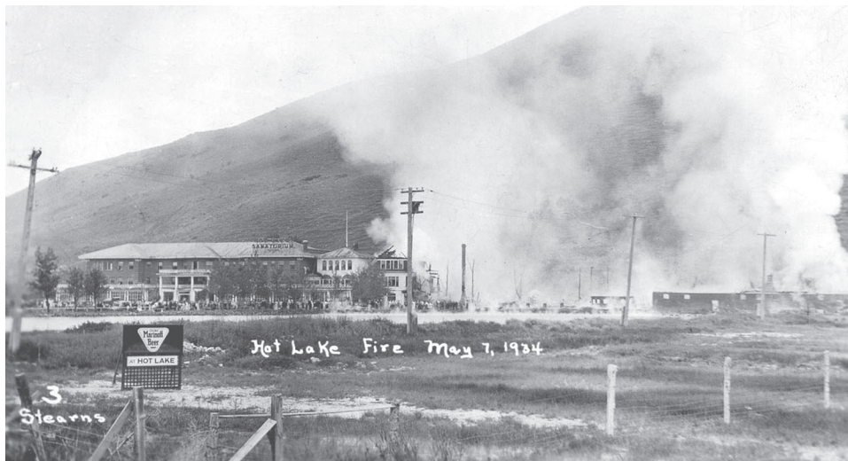
Fire at Hot Lake Sanatorium destroyed wooden structures Photo by Mae Stearns, 1934
